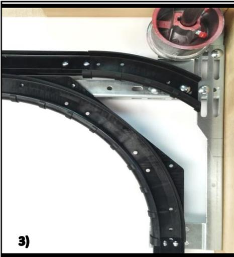
Install the door same as it would be for standard headroom fixing the horizontal tracks to ceiling before sliding in the top, low headroom track
